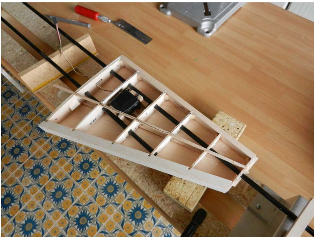
Figure 57: Verify servo position and covering panels.
