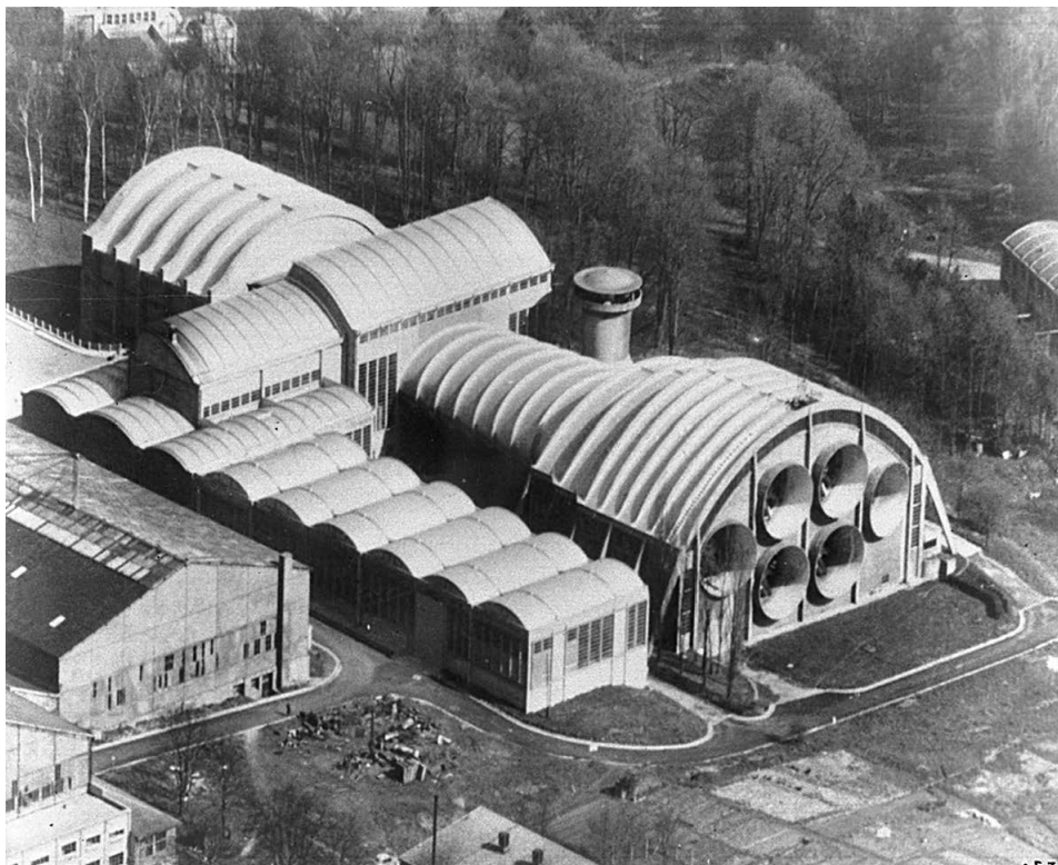
Figure 2.10 View of the large S1Ch wind tunnel in Meudon [20].
