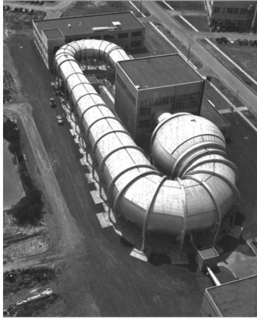
Figure 2.21 The 12-foot pressure tunnel with several angular stages. The spherical bulge houses the antiturbulence screens [19].
