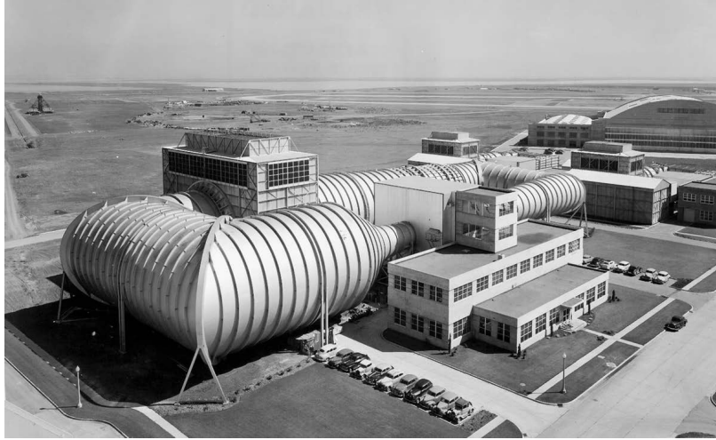
Figure 2.18 The Ames 16-foot wind tunnel [19].
