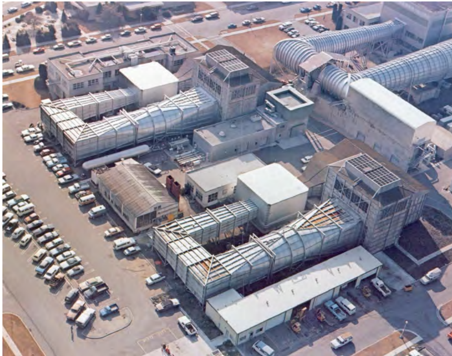
Figure 2.17 The two wartime 7 \times 10 foot wind tunnels built at Ames [19].
