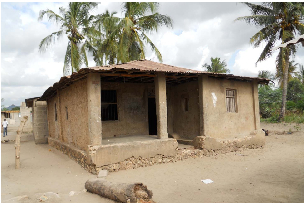
Figure 31 - Raised foundation with stone bricks and mortar (photo by R. De Risi)
