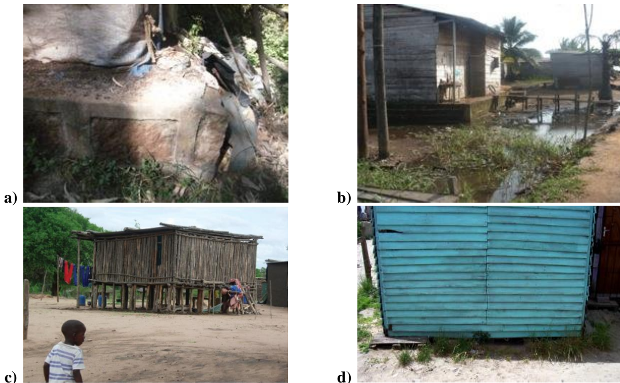
Figure 8 – Various types of raised foundation: (a) raised foundations made up of cement-stabilized earth and stone (Little Akaki, Addis Ababa, Photo by F. Jalayer); (b) construction of brick perimeter walls (Mbanga, Douala, Figure by R. Fuemba); (c) stilt foundations (Chicualacula, Mouzambique, figure courtesy of (Feuerhake 2010)); (d) use of pallets (Lotus river, South Africa, figure courtesy of (Bouchard 2007));
