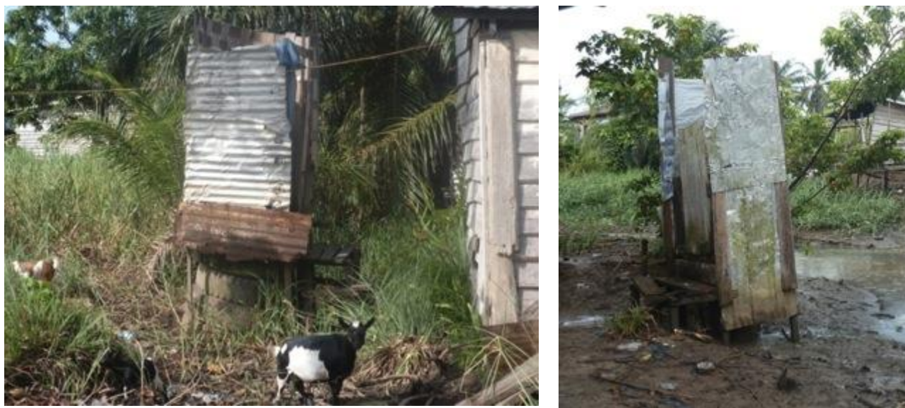
Figure 11 – Examples of latrines not elevated properly (Mbanga, Douala, photos by R. Fuemba)
