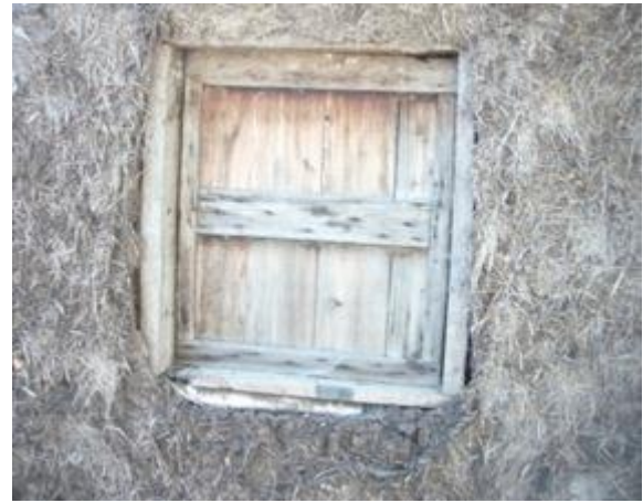
Figure 13 – (a) a sealed window in a mud and wood wall protected by plastic sheets; (b) a non water proof window in an un-protected mud and wood wall (Little Akaki, Addis Ababa, photos by F. Jalayer)
