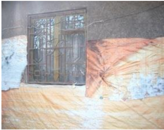
Figure 13 – (a) a sealed window in a mud and wood wall protected by plastic sheets; (b) a non water proof window in an un-protected mud and wood wall (Little Akaki, Addis Ababa, photos by F. Jalayer)
