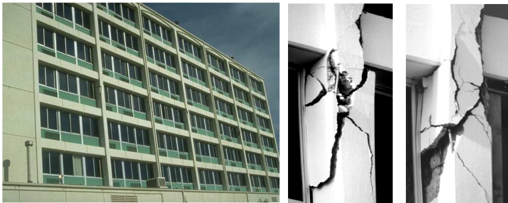
Figure 1.1: (a) Holiday Inn hotel building [56] and (b) photos of the damages in the building after Northridge earthquake, 1994, in the longitudinal direction [57].
