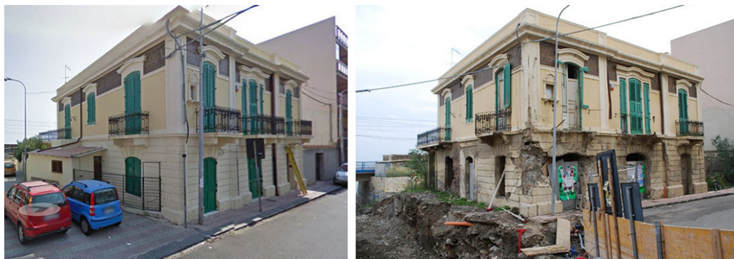
Fig. 5-4: Building before and after the event of October 2009.
