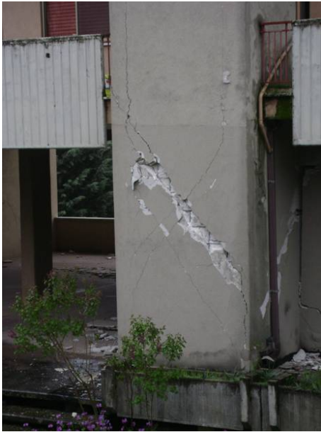
Figure 7.13. Failure in reinforced concrete walls.
