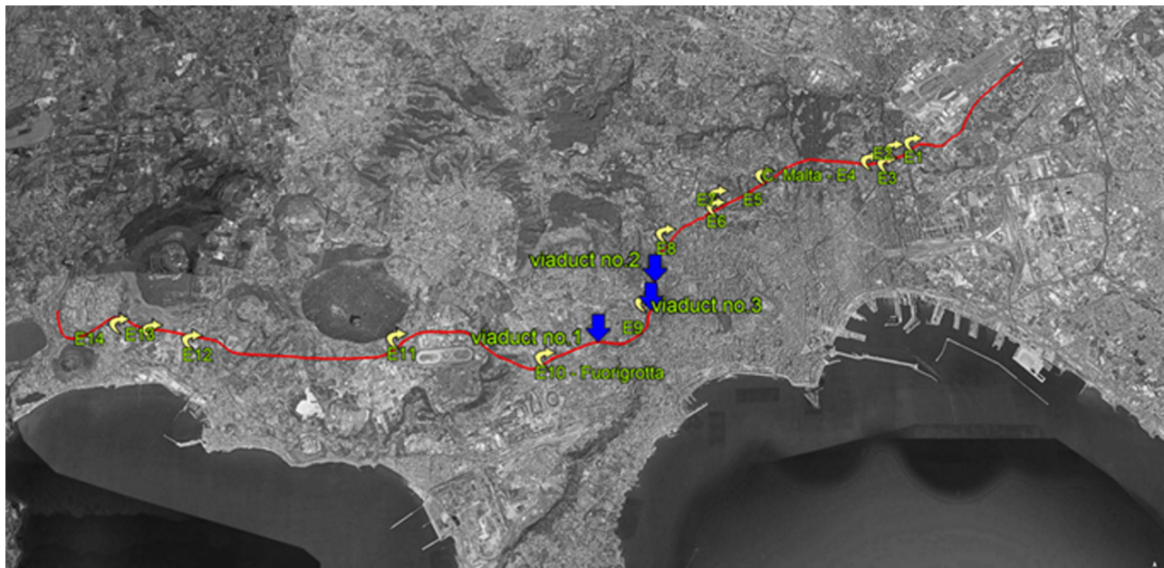
FIGURE 2 Layout of the A56—Tangenziale di Napoli—road network, with its 14 junctions and the three viaducts considered herein labeled
