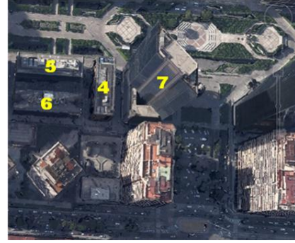
Fig. 3: aerial optic view of analyzed buildings
