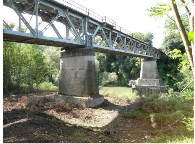
Fig.2 Picture of the bridge.
