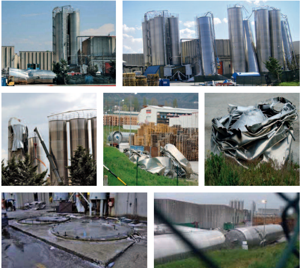
Fig. 7 Pictures of the sili after the seism. Photo by G. Verderame, ISPRA, F.M. Mazzolani.
