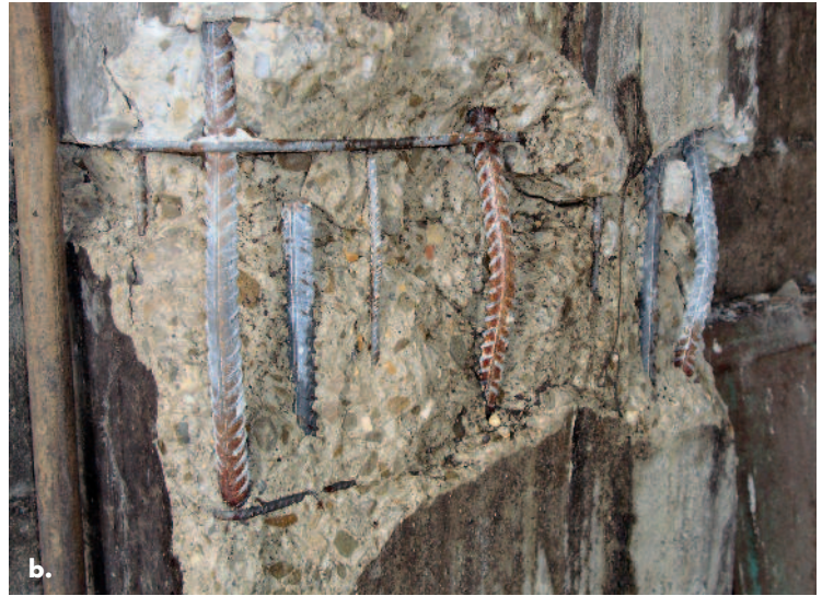
Fig. 1 Plastic hinge in columns of industrial buildings: (a) FIAT garage at Pile; (b) building used for bovine-breeding at Fossa.
