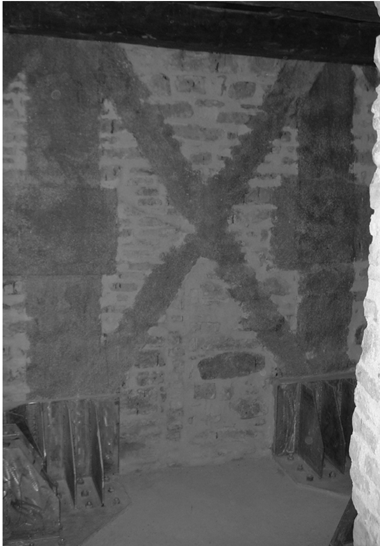
Figure 4. Installed composites and base anchorage.
