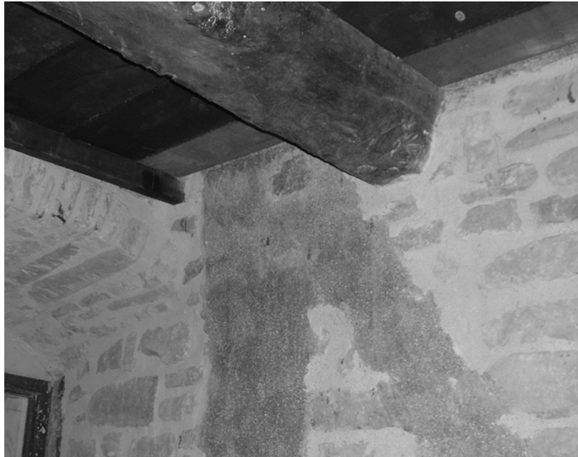
Figure 6. Composites near to unremoved wooden floor.
