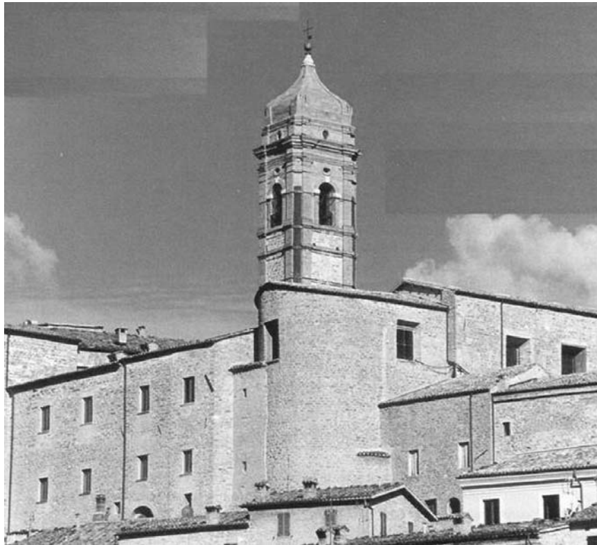
Figure 8. Bell tower after intervention.
