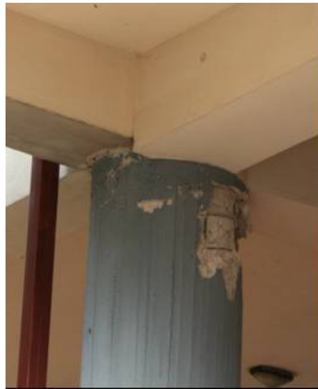
Figure 7.9. Column with smooth bars and poor transversal reinforcement (a); damage to a column due to axial force and bending moment (b)
