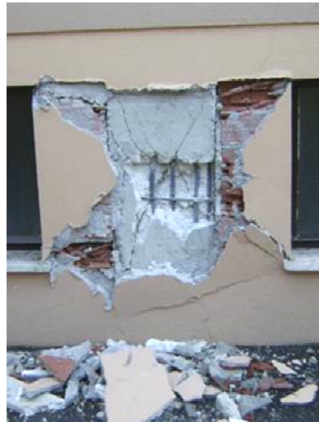
Figure 7.11. Shear failure of: (a) column adjacent to partial infilling panels, (b) squat column adjacent to basement level concrete walls
