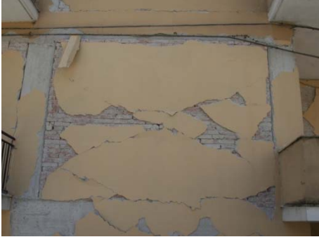
Figure 7.16. Infill panel failures: diagonal cracking (a), and corner crushing (b) mechanisms.
