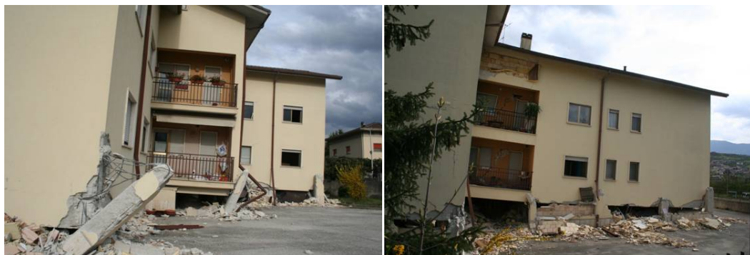
Figure 7.21. Building collapse mechanism. Damage along South-East (a) and South-West (b) wings of the building (Verderame et al., 2009).
