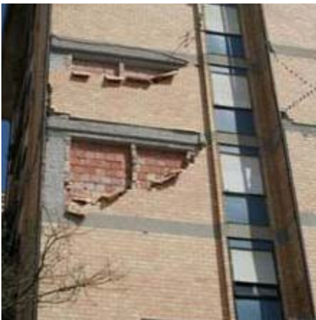
Figure 7.17. External infill panel failures without connection between layers (a) and with ineffective connection (b).
