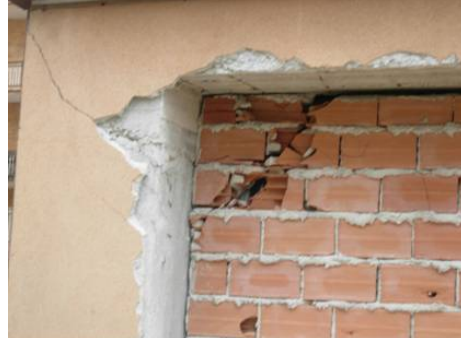
Figure 7.16. Infill panel failures: diagonal cracking (a), and corner crushing (b) mechanisms.
