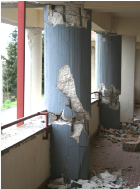
Figure 7.11. Shear failure of: (a) column adjacent to partial infilling panels, (b) squat column adjacent to basement level concrete walls
