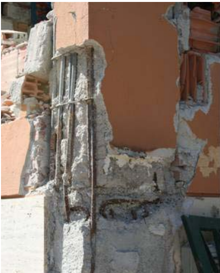
Figure 7.9. Column with smooth bars and poor transversal reinforcement (a); damage to a column due to axial force and bending moment (b)
