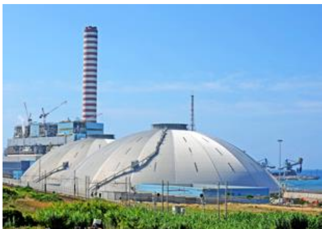
Fig. 5 coal-fired power plant near Civitavecchia Port
