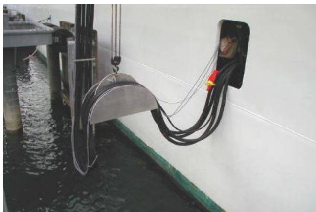
Fig. 2 Cold ironing arrangement in Juneau (Alaska)-1-
