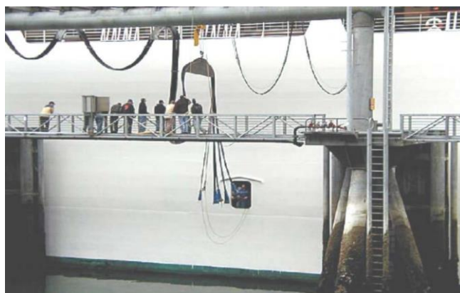
Fig. 3 Cold ironing arrangement in Juneau (Alaska)-2-
