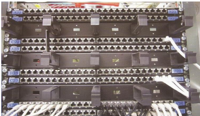
Patch panel for UTP cables: front view
