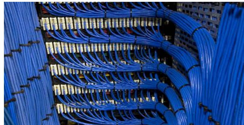
Patch panel for UTP cables: rear view
