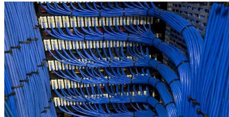
Patch panel for UTP cables: rear view
