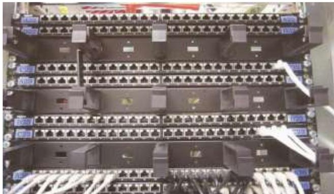
Patch panel for UTP cables: front view
