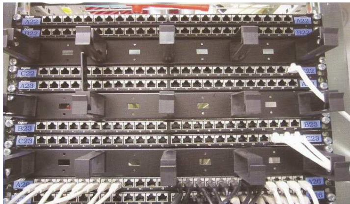
Patch panel for UTP cables: front view
