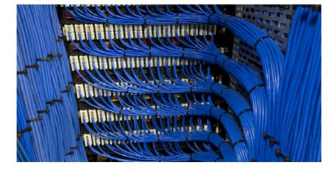
Patch panel for UTP cables: rear view
