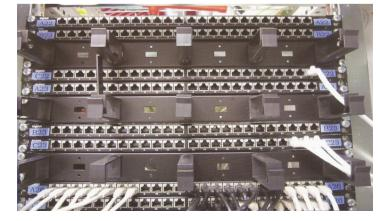
Patch panel for UTP cables: front view
