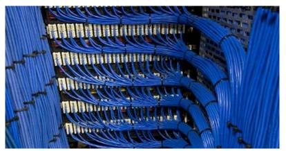
Patch panel for UTP cables: rear view
