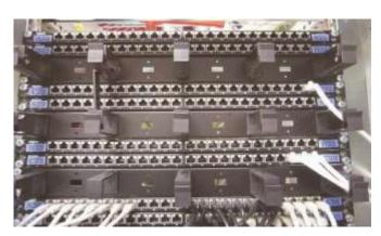
Patch panel for UTP cables: front view
